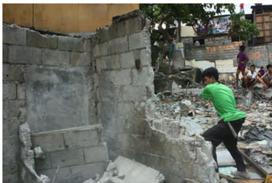
Clearing Demolition at Corazon de Jesus, San Juan City
